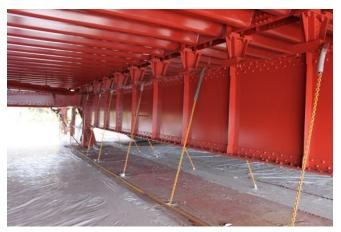
elements, and building up the fresh layers of paint to defend the structure against the salty marine air for decades to come. Bridge forces have completed the initial phase of the project which refurbished the southernmost three girder spans of the Bridge and continue working northward on the truss span sections approaching the Fort Point Arch.
