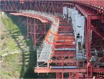
Contractors also continued to remove and replace the west sidewalk handrail in FY 20/21 as part of the Wind Retrofit Project. Most noticeably, the new handrail features thinner vertical slats than the old handrail, along with other design elements to reduce wind drag, while blending in with the existing Bridge. Contractors completed installing the new handrail in late 2020.
