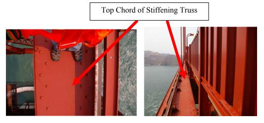
The maximum distance that personnel will have to walk along the truss top chord is 75 feet, since the gates are spaced 150 feet apart. The suspender ropes are spaced 50 feet apart, so there will be instances where workers will need to climb around the outside of the suspender ropes as they walk along the top chord to the travelers. There will also be instances where workers will need to climb around the belvederes on the traveler rail as discussed above.
