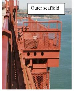
or other such support when accessing the outer scaffold. To aid in the movement of workers over the top of the railing, step ladders designed specifically to attach to the outside hand rail top members are used.
