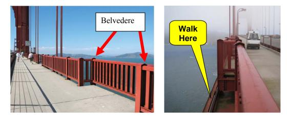
Fall protection will be required when walking from the gates to the travelers. It is proposed that a permanent stainless steel safety cable be installed on the outboard side of the east and west outside handrail or new barrier, along the entire length of the Bridge, for workers to "tie-off" to when walking along the stiffening truss upper chord or traveler rail. The cable will be on the outer face of the outside hand rail posts to minimize its visibility.
