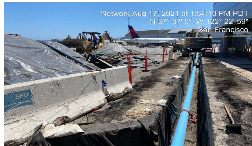
Sample water line installation from Contract 10010 (2021).
