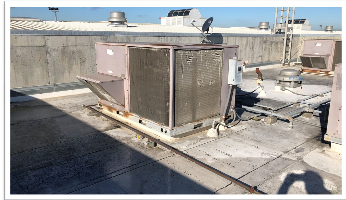
Typical Rooftop Gas Fired/Electric Packaged AC Unit to be replaced with New Packaged Heat Pump
