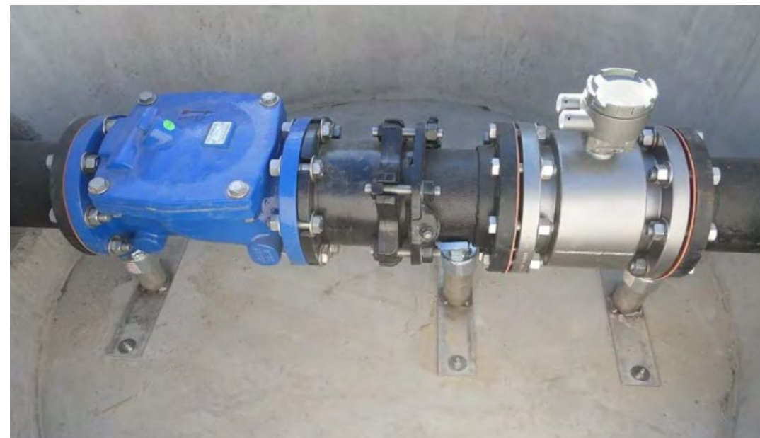
Flow Sensor Installed in Vault
