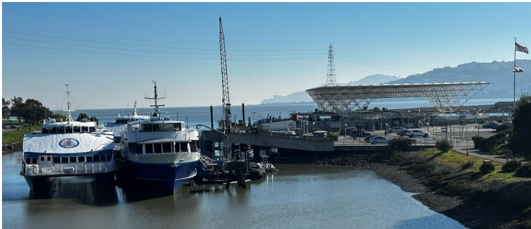
Figure 3. South view of Berth 3, Berth 2 and the Larkspur Ferry Terminal Building in the background
