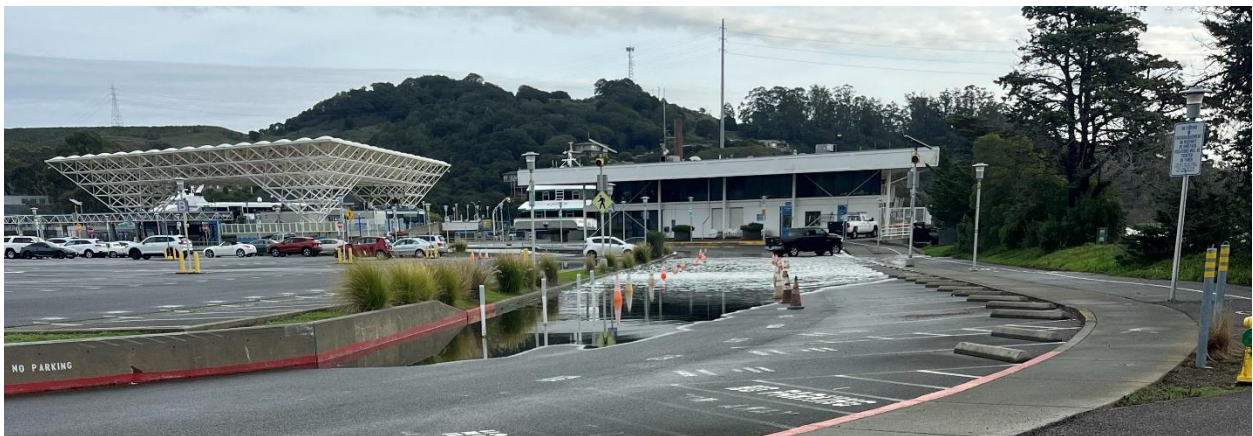
Figure 19. Flooded area in the southern section of the Larkspur Ferry Terminal access road on January 2, 2026, at 9:39 AM, TWL = 8.31 feet NAVD88 (NOAA 2025b)
