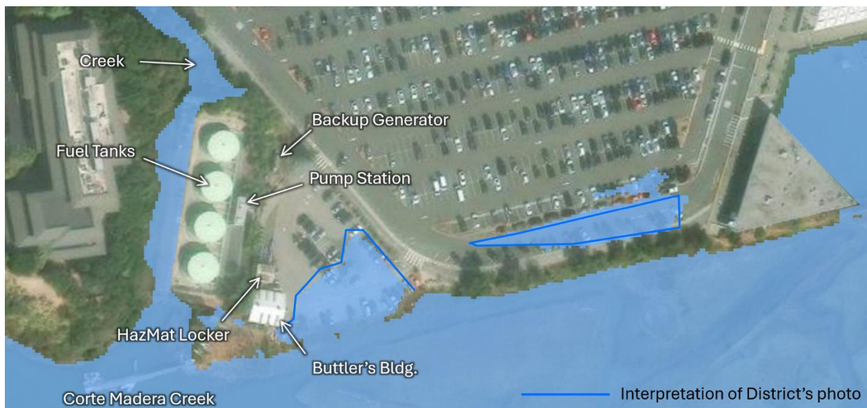
Figure 25. Flooded area in the Butler Building area and southern section of the Larkspur Ferry Terminal access road according to the NOAA DEM on January 4, 2026, at 12:12 PM, TWL = 8.23 feet NAVD88 (NOAA 2025b)
