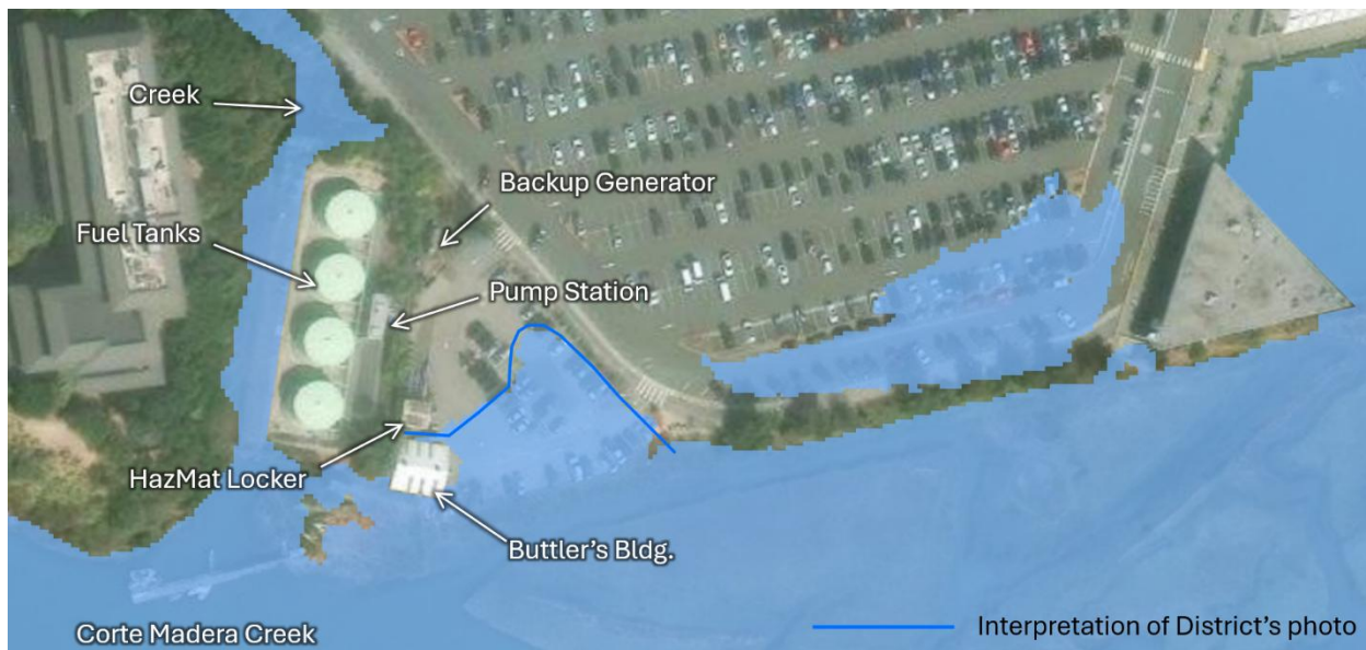
Figure 22. Flooded area in the Butler Building area and southern section of the Larkspur Ferry Terminal access road according to the NOAA DEM on January 3, 2026, at 10:36 AM, TWL = 8.73 feet NAVD88 (NOAA 2025b)
