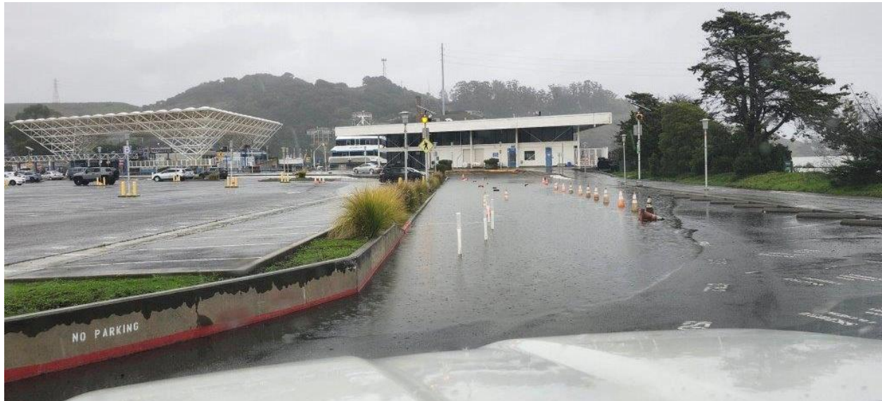
Figure 24. Flooded area in the southern section of the Larkspur Ferry Terminal access road on January 4, 2026, at 12:12 PM, TWL = 8.23 feet NAVD88 (NOAA 2025b)
