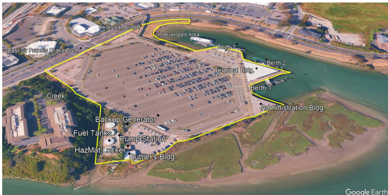
Figure ES-1. Aerial view of the Larkspur Ferry Terminal, key locations and perimeter inspected (image source: Google Earth Landsat/Copernicus)
