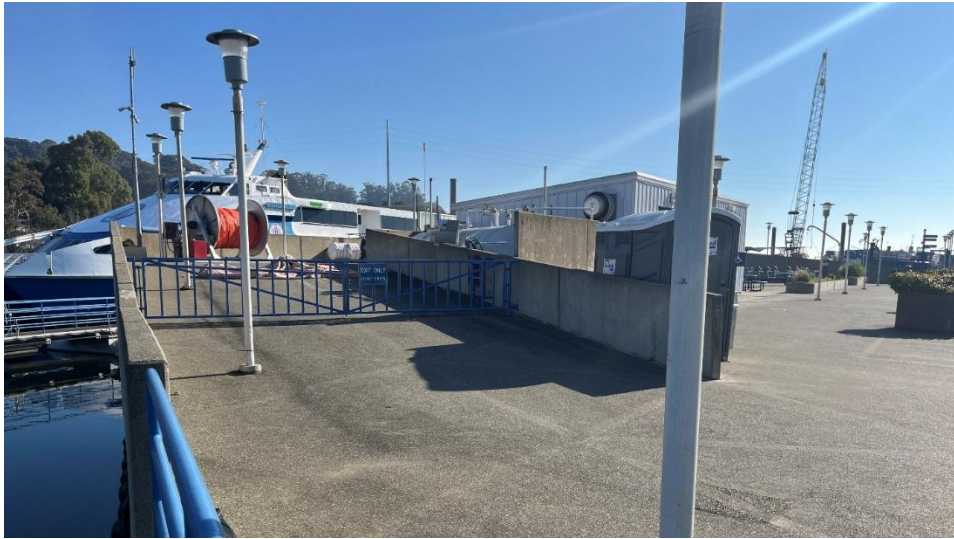
Figure 2. East view of Berth 3
