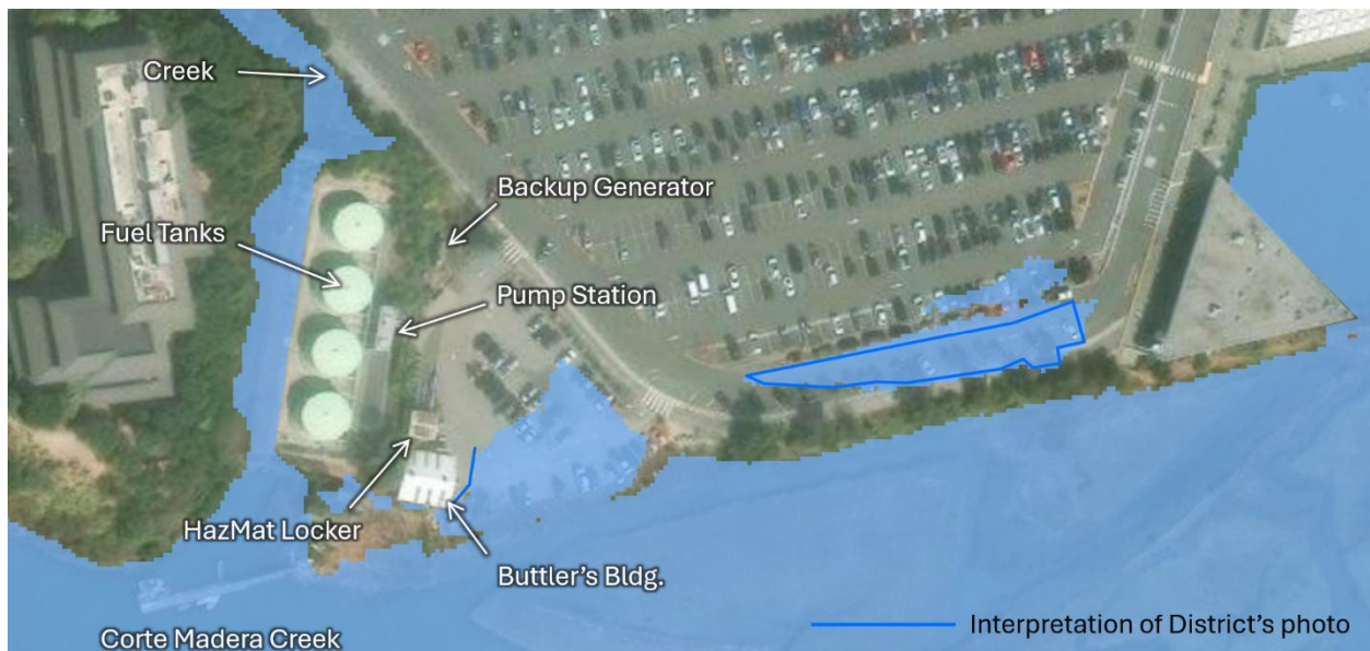
Figure 20. Flooded area in the Butler Building area and southern section of the Larkspur Ferry Terminal access road according to the NOAA DEM on January 2, 2026, at 9:39 AM, TWL = 8.31 feet NAVD88 (NOAA 2025b)
