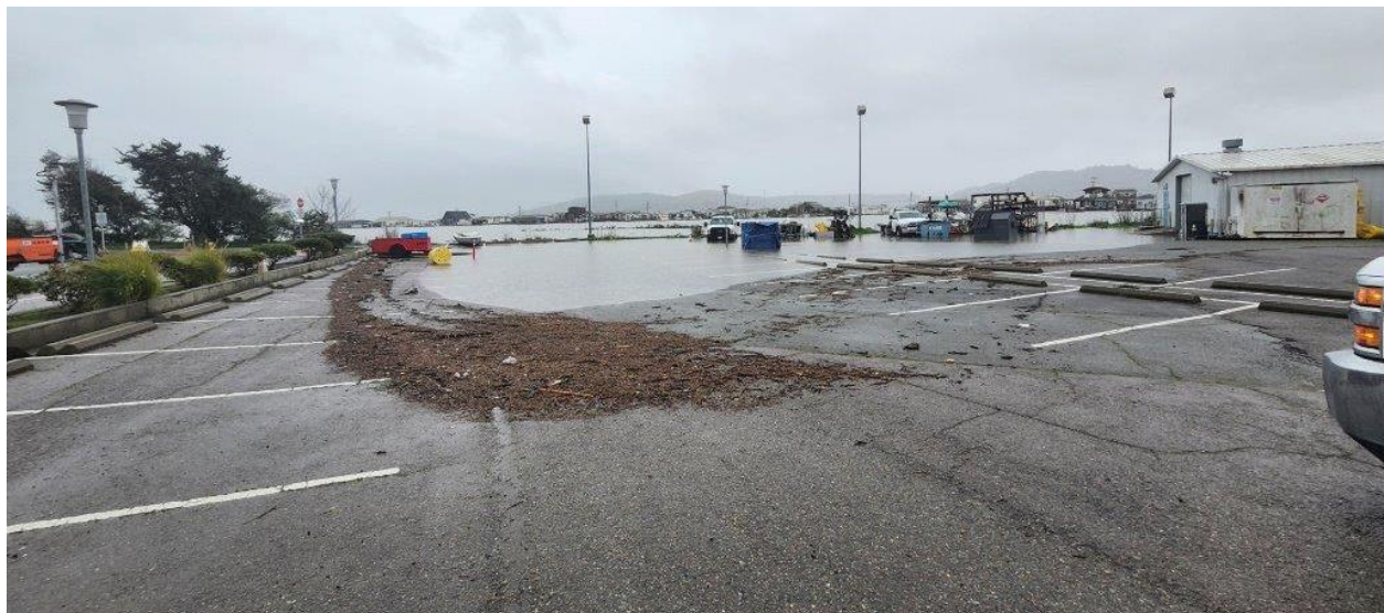
Figure 21. Debris in the employee parking lot in the Butler Building area marking the edge of the highest floodwater elevation on January 3, 2026, at 10:36 AM, TWL = 8.73 feet NAVD88 (NOAA 2025b)
