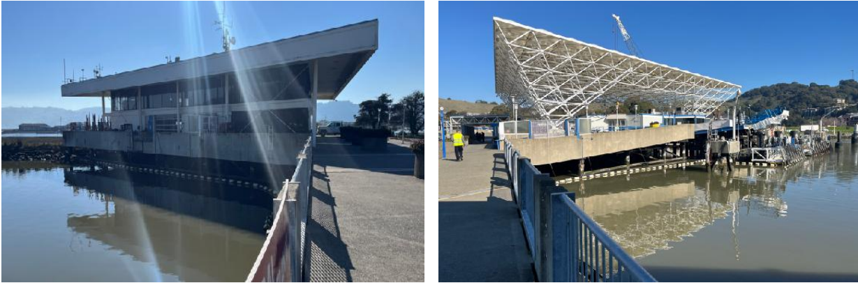
Figure 15. Southwest view the Administration Building (left) and northeast view of Larkspur Ferry Terminal Building Berth 1
