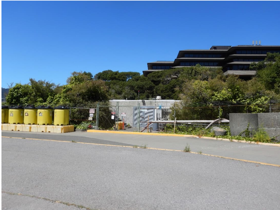
Photograph 14: View of the underground pump station and utilitarian steel tanks that are hidden from view, facing west (Jacobs 06/04/2021).
