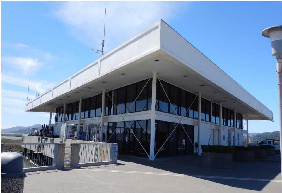
Photograph 8: View of the Service Building, facing south (Jacobs 06/04/2021).
