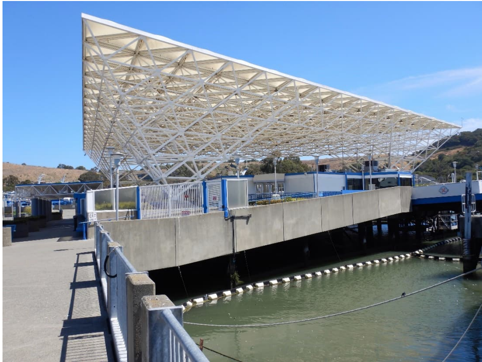
Photograph 10: View of the loading platforms located around the Shelter Building, facing north (Jacobs 06/04/2021).
