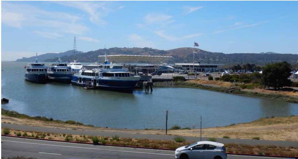
Photograph 2: View of the Larkspur Ferry Terminal, facing south (Jacobs 06/04/2021).
