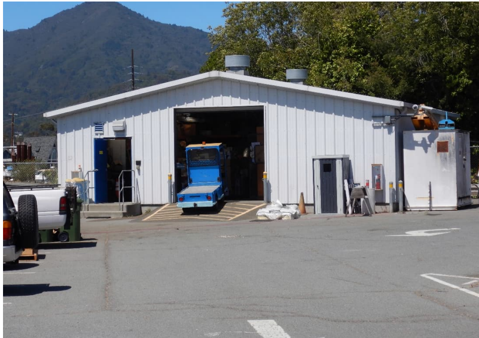
Photograph 13: View of the Utility Building in the Maintenance Yard, view west (Jacobs 06/04/2021).
