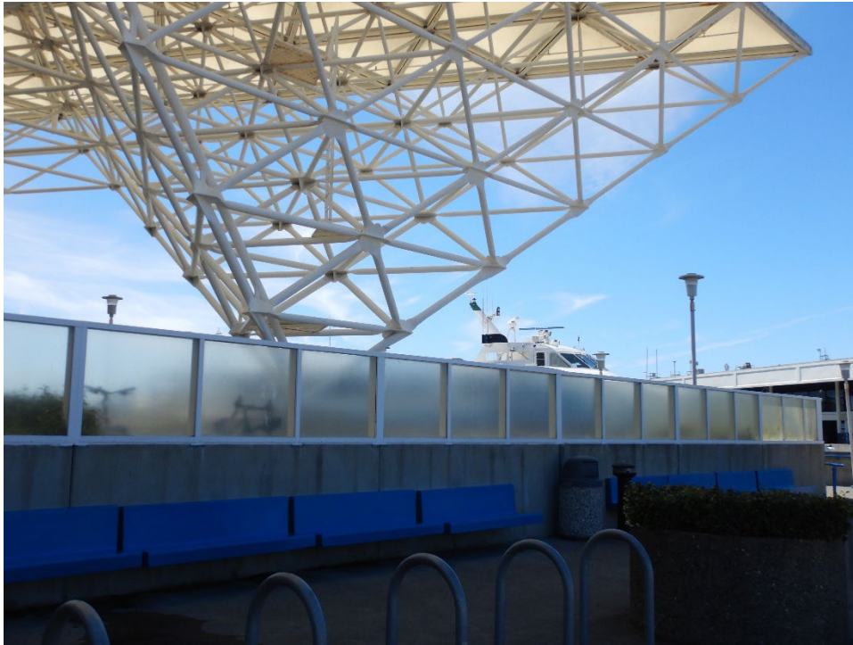
Photograph 3: Detail of southwest base support, facing south.
