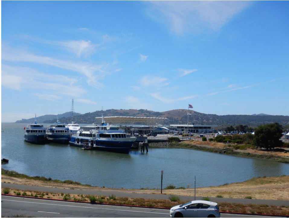
Photograph 1: Overview of Larkspur Ferry Terminal, facing southwest.
