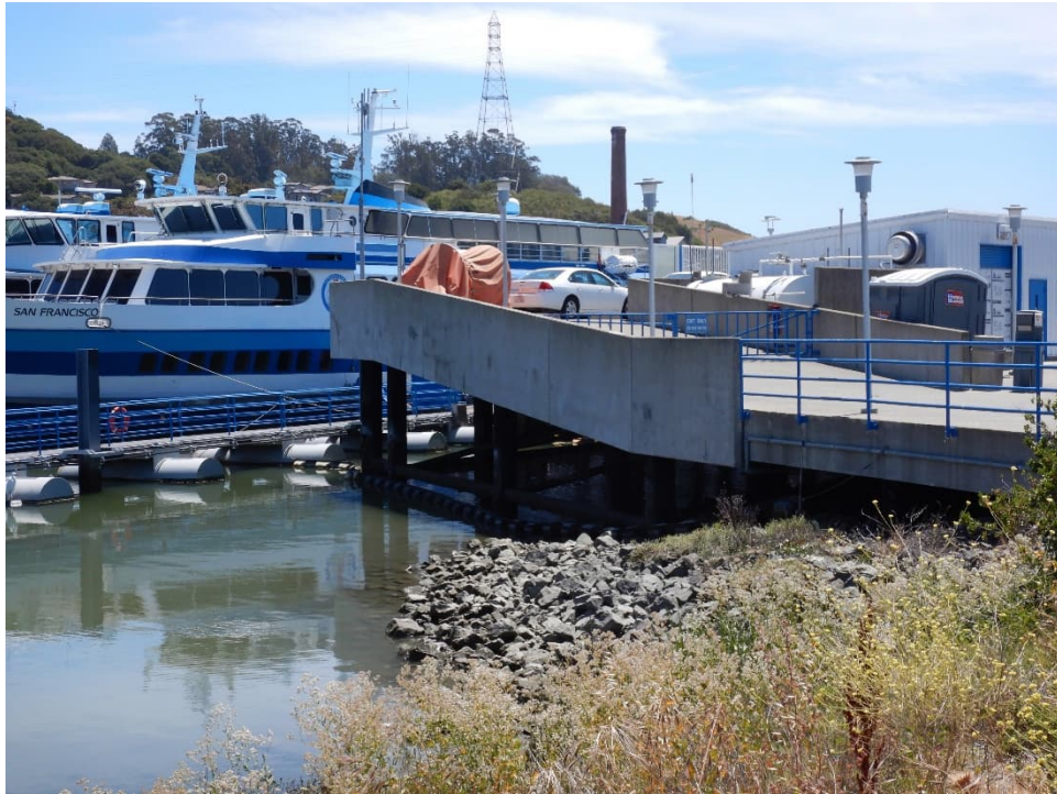
Photograph 12: View of the Shed Building and the run-up platform, view east (Jacobs 06/04/2021).
