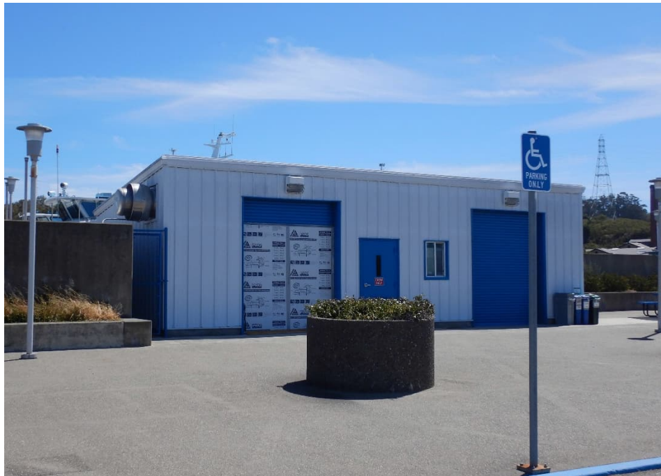
Photograph 11: View of the west façade of the Shed Building (Jacobs 06/04/2021).
