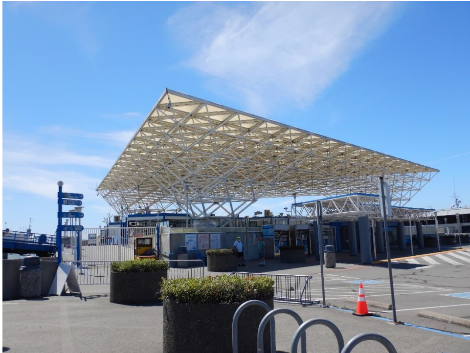
Photograph 4: View of the northeast and west sides of Shelter Structure, facing south (Jacobs 06/04/2021).
