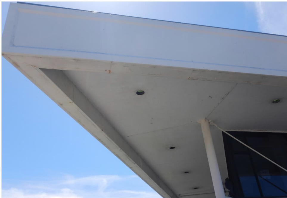
Photograph 9: View of the sheet metal fascia of the Service Building, facing south (Jacobs 06/04/2021).
