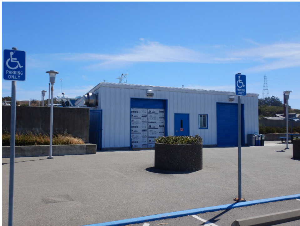
Photograph 8: Utility shed, facing east.
