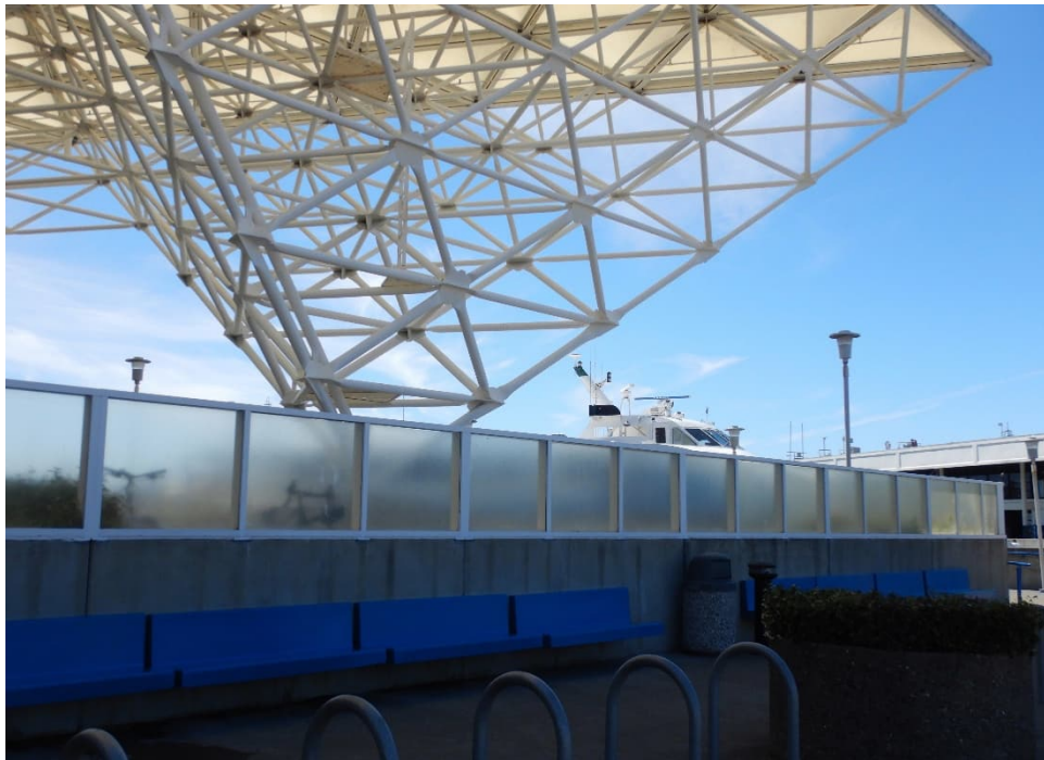
Photograph 5: Concrete pyramidal base supports of the Shelter Structure, facing east (Jacobs 06/04/2021).
