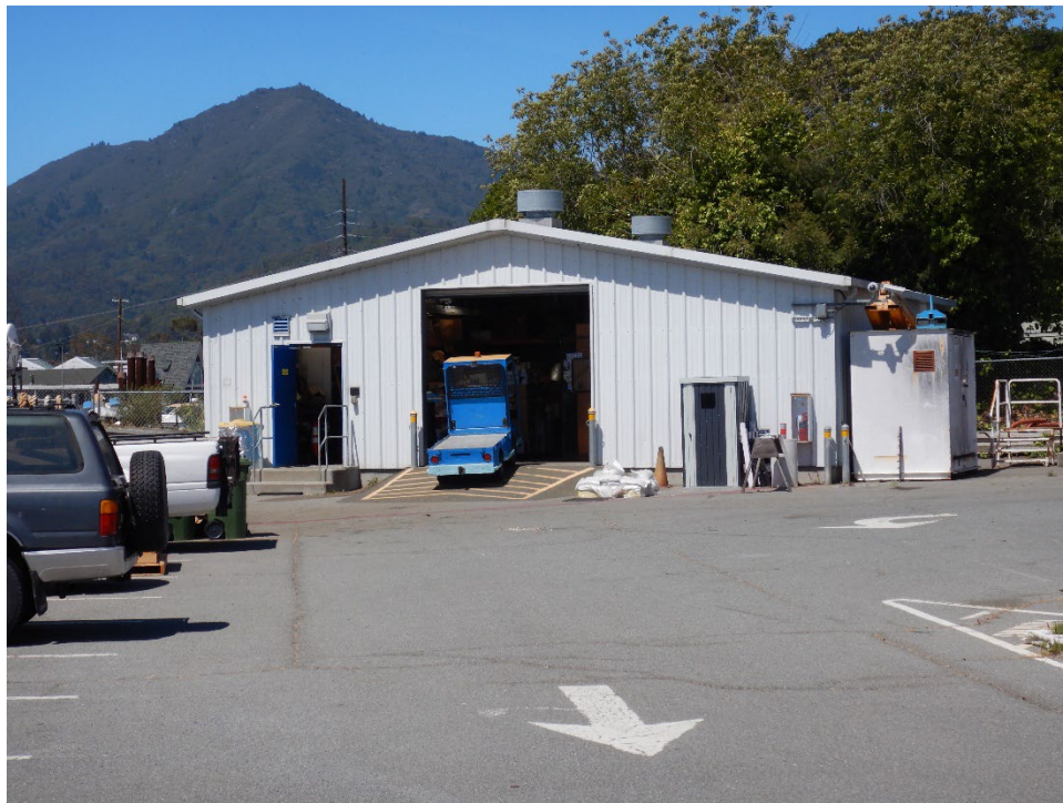
Photograph 10: Maintenance Yard, facing southwest.
