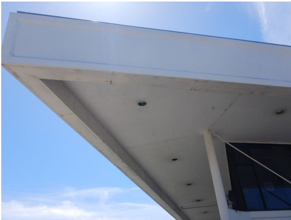
Photograph 6: Service Building eave detail view, facing south.
