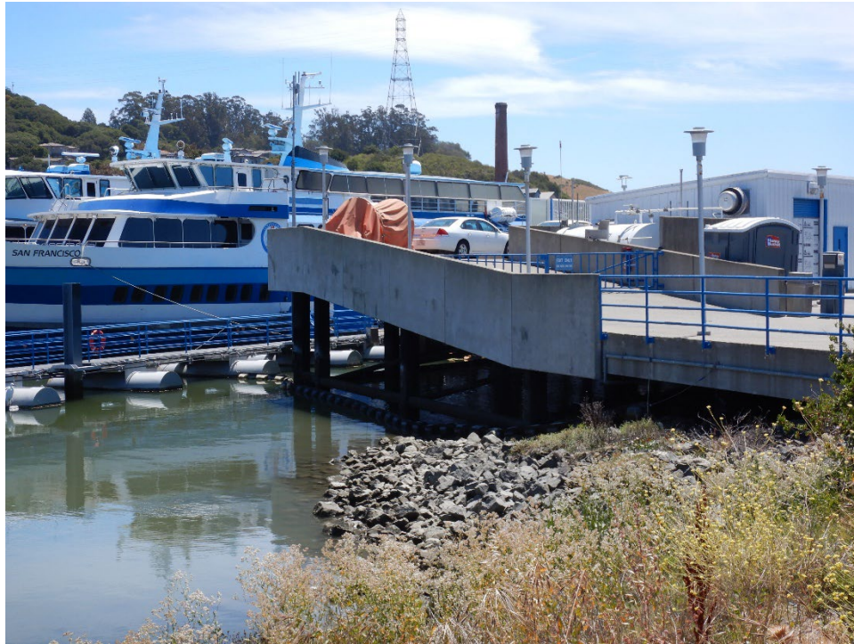
Photograph 9: North Landing Structure, facing south.
