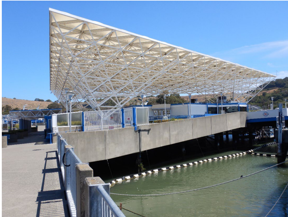
Photograph 7: View of piling supports for Shelter Structure and loading platforms, facing north.
