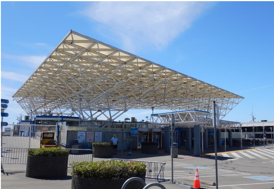
Photograph 7: View of Larkspur Ferry Terminal, with smaller spaceframe awning on the west elevation visible, facing east (Jacobs 06/04/2021).
