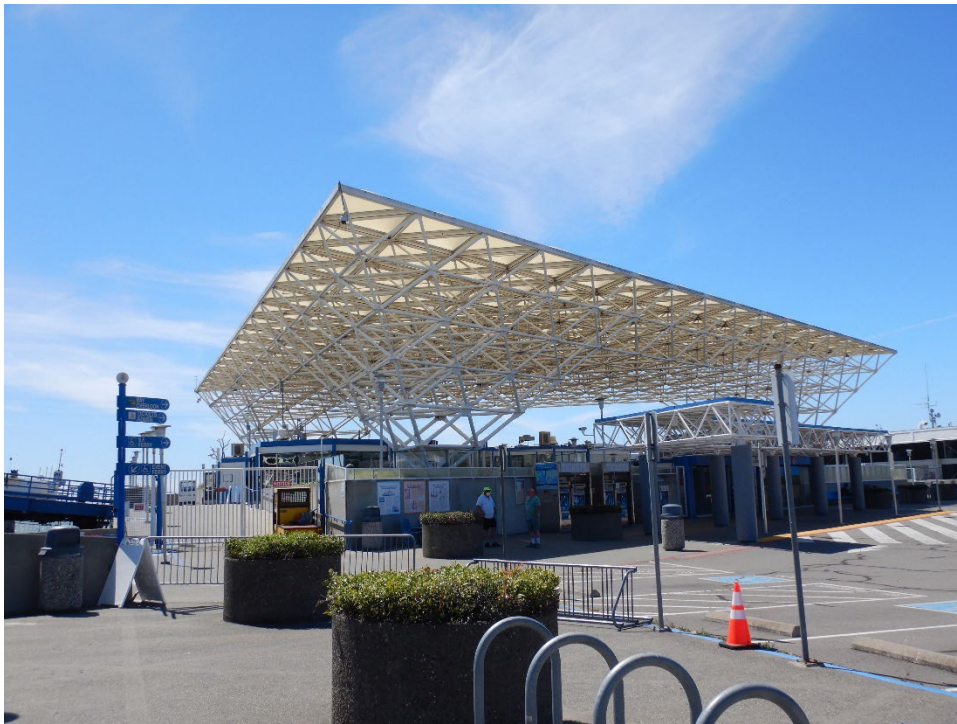
Photograph 2: Shelter Structure, facing southeast.
