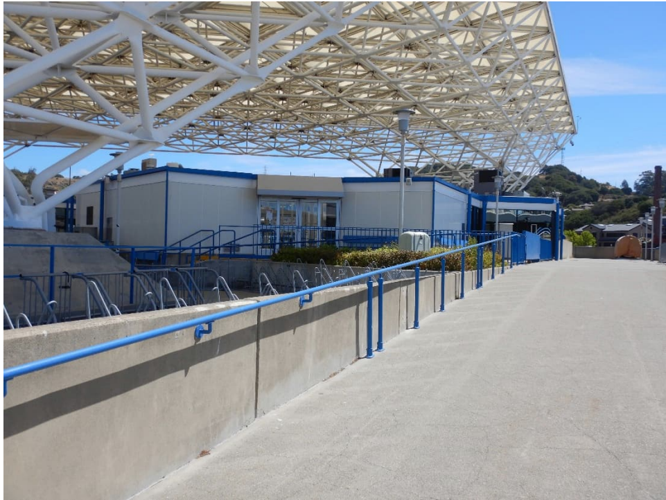
Photograph 6: View of the kiosks, facing northeast (Jacobs 06/04/2021).
