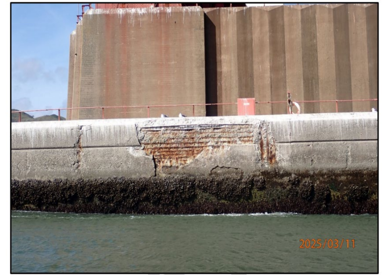
Photo 23 – South Tower Pier Fender, South Face, Spalling with Exposed Reinforcing
