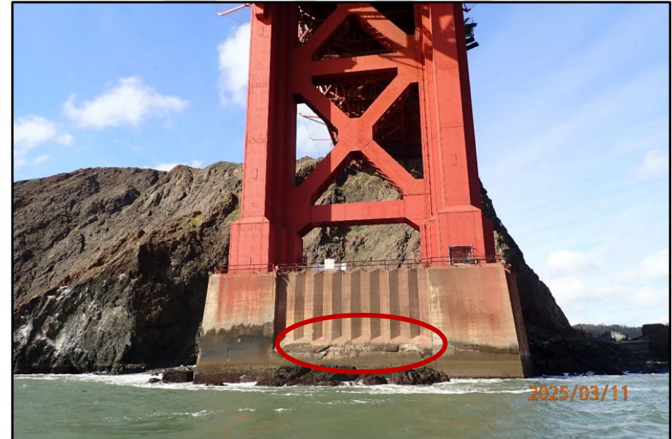
Photo 26 – North Tower Pier, South Face, Rock Outcropping to Left (West Face) and In Foreground (South Face), Spalling with Exposed Reinforcing Above MHHW
