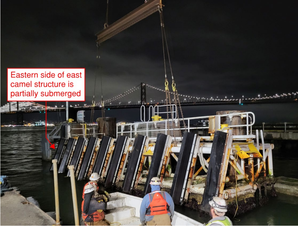
Figure 1-East Camel structure shown listing prior to crane lift
