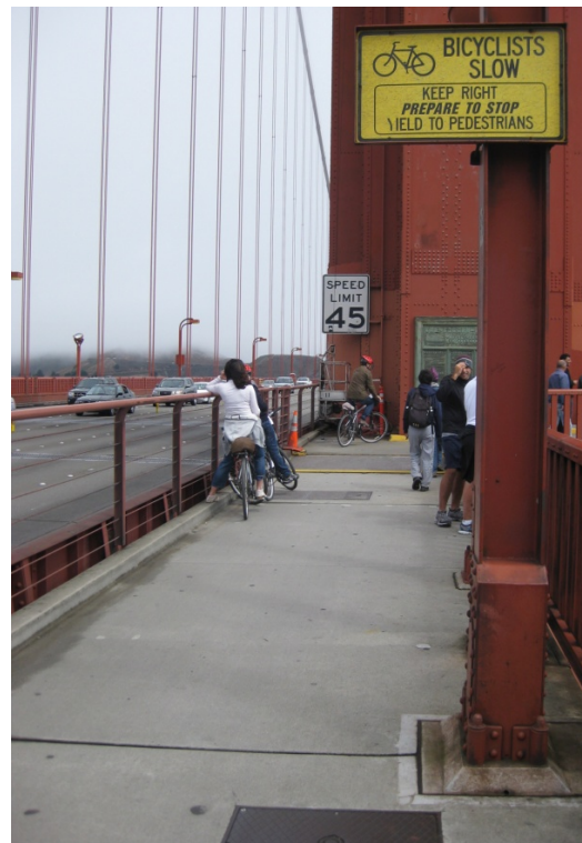
Figure 19: Existing Bicycle Sign on the Bridge Towers
