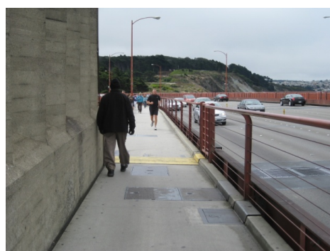
Figure 1: A narrow section of the sidewalk adjacent to a pylon on the east side
