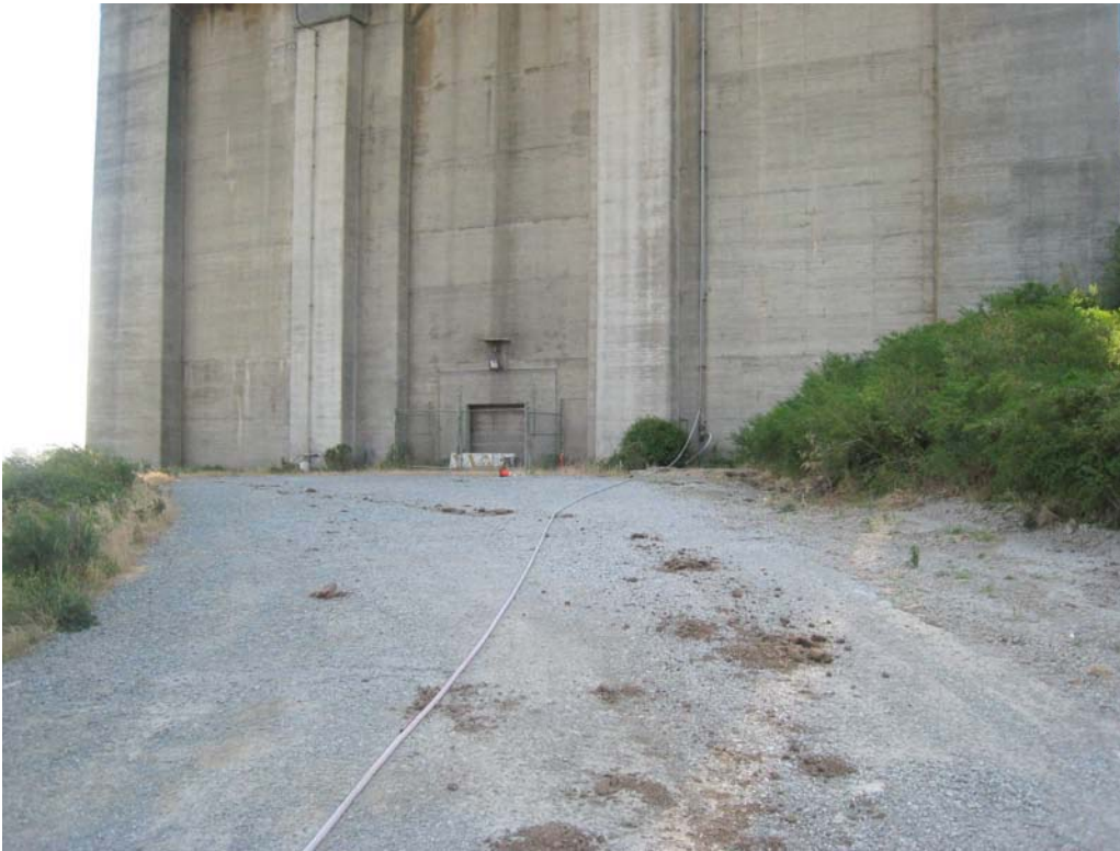
Staging Area 3 (upper area.); located within GGNRA, south of lower area
