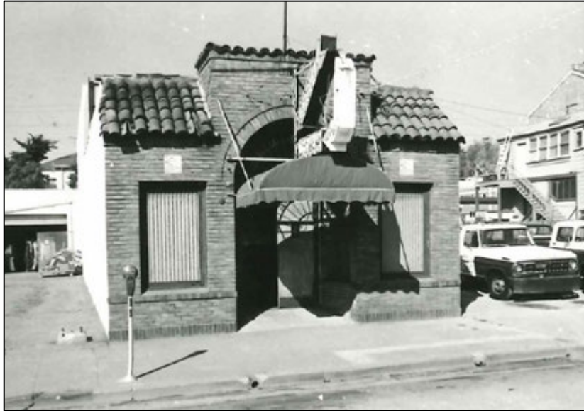
Figure 2. View of east (Primary) façade, facing west. Source: Charles Hall Page & Associates, Inc 10/11/1976.
