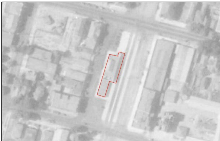
Figure 2. Aerial photograph showing the footprint of NWP Railroad Depot, 1931; visible are the passenger waiting room (with raised, gabled roof), passenger arcade facing the tracks, and south warehouse wing. Source: University of California, Santa Barbara Library (Flight C_1595, Frame 28), edited by ICF.
