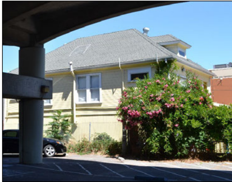
Figure 2. View of west façade, facing east. Source: ICF 8/11/2020.
