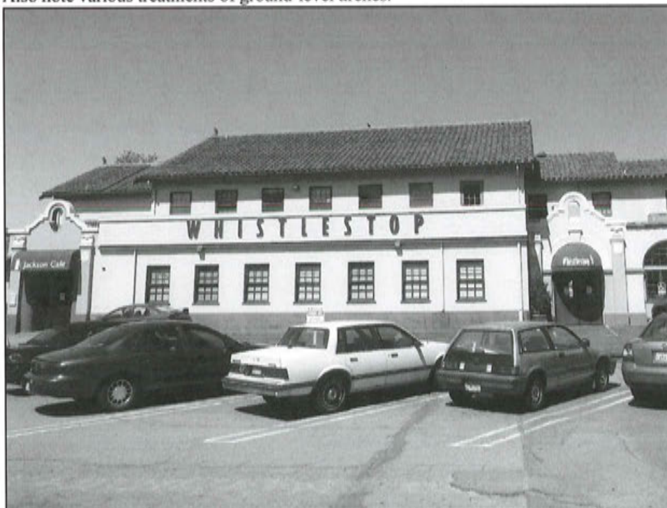
Photograph 6: Mid-section of east side. 1985 second-story addition above 1939-1946 addition, camera facing west.
