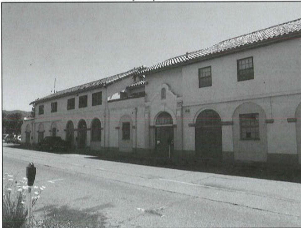
Photograph 4: West side of the building, camera facing northeast. Note second-story addition, parapet flush with addition, and various treatments of ground-level arches.
