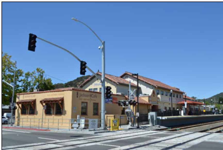
Figure 9. South and east façades, viewed facing northwest.
