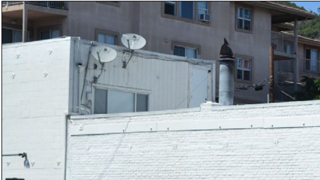
Figure 4. View of east of façade of two-story residential addition, facing west. Source: ICF 8/11/2020.
