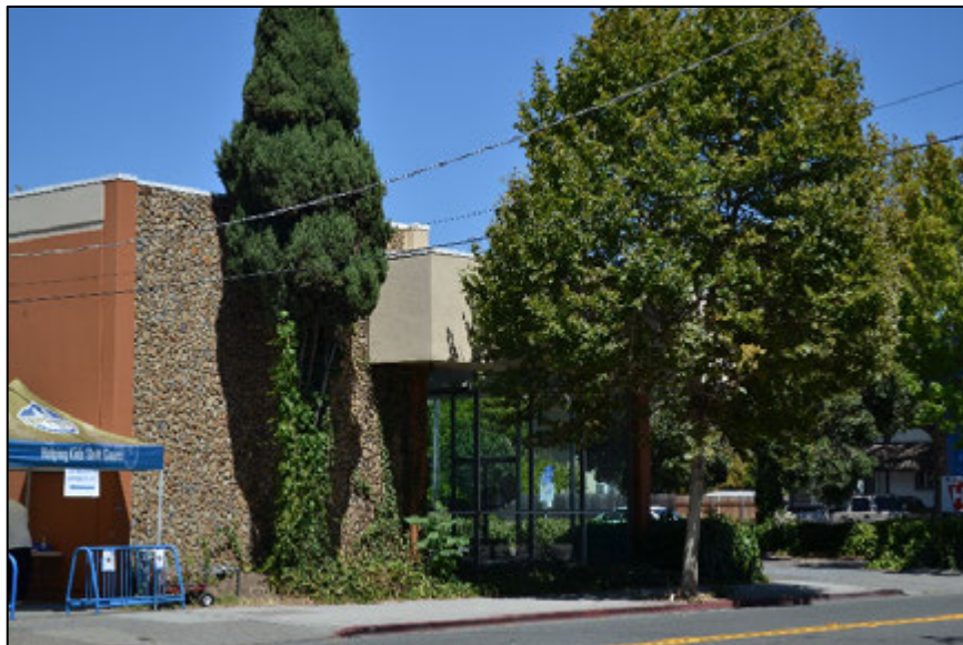
Figure 3. View of south façade, facing northeast, showing the stone veneer cladding and glazed showroom. Source: ICF 8/11/2020.
