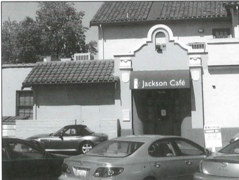
Photograph 8: Southernmost entry on east side, camera facing west.
