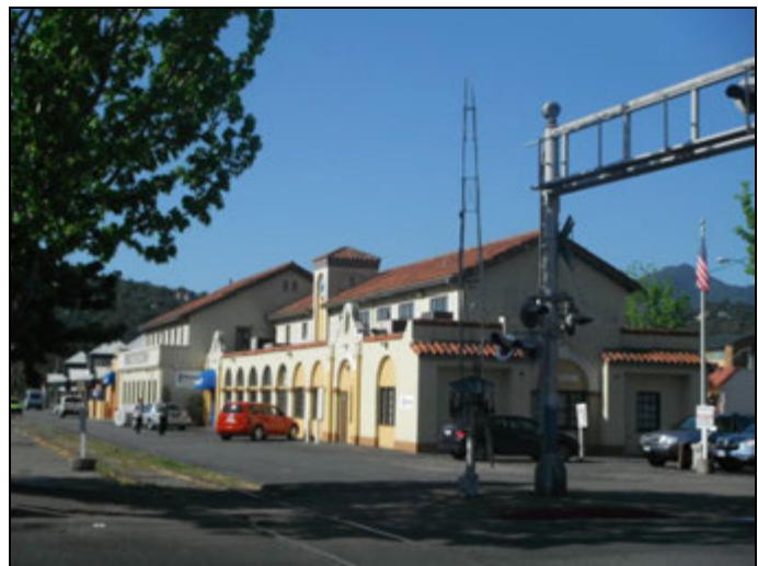
Photograph 6. Northwestern Pacific Depot. 930 Tamalpais Ave. View southwest.
