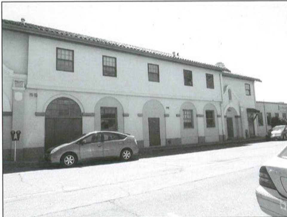
Photograph 5: West side showing 1985 second-story addition, camera facing southeast. Also note various treatments of ground-level arches.
