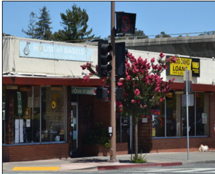
Figure 4. View of primary (south) façade, showing brick cladding and cedar shingle siding, facing northeast. Source: ICF 8/11/2020.
